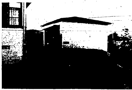
Now you see this garage in Pacific Palisades, Calif. ...
