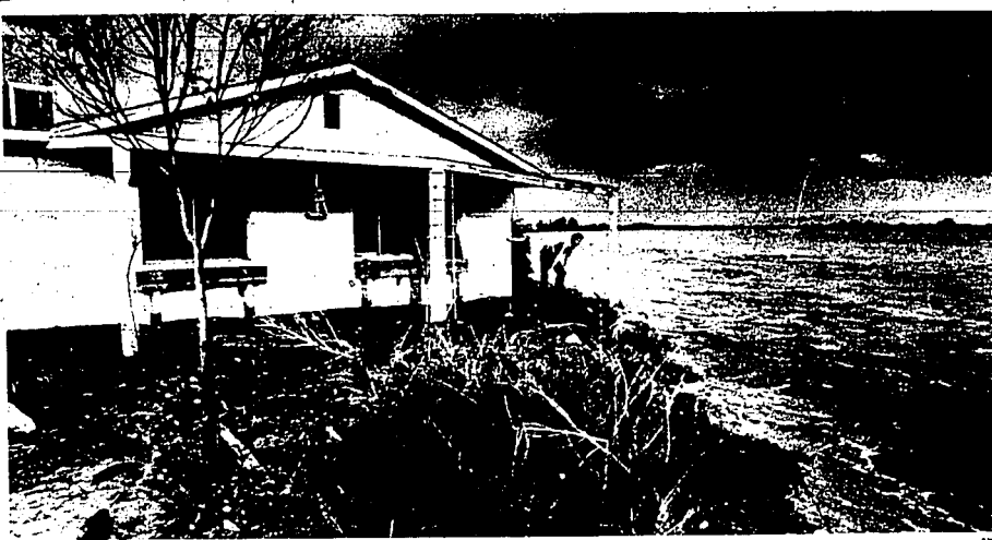
Deputy sheriff inspects riverfront home during high water in Phoenix as Feb. 16 flood raged
