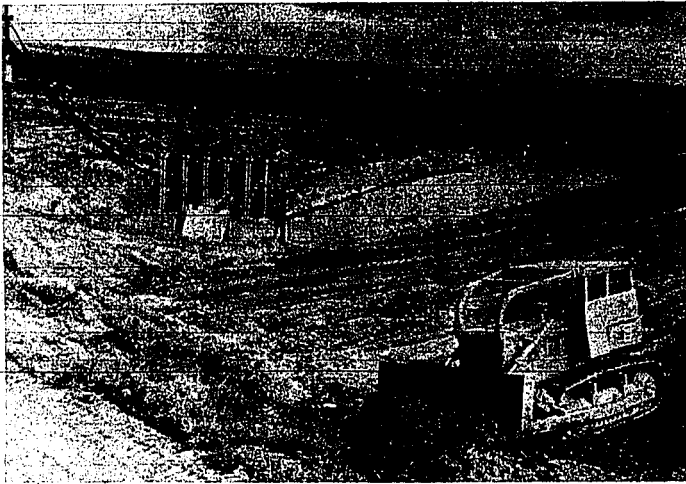
Bulldozer repairs erosion damage to drainage canal on Bell Rapids Irrigation system
