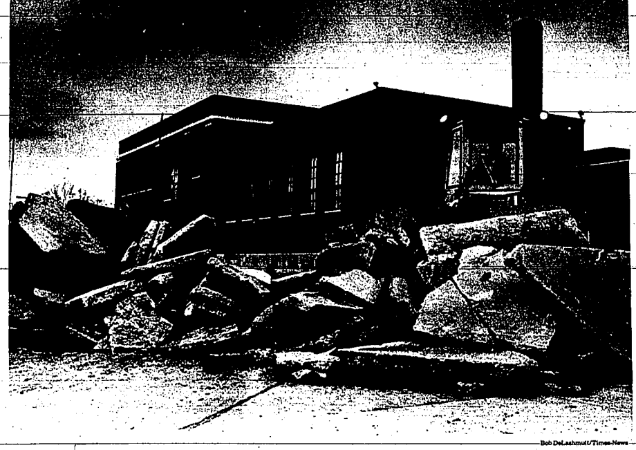
Clearing the way
