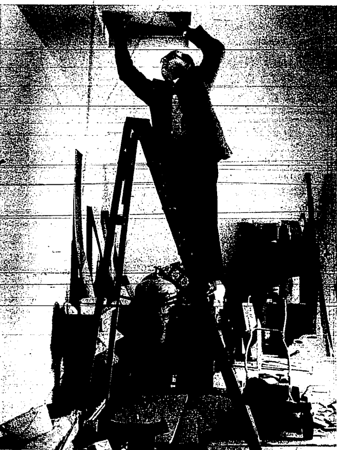
Twin Falls Building Inspector Clare Harkins checks insulation depth in attic Wednesday
