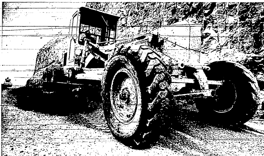
Construction crews this week finished smoothing Canyon Springs Road, closed weekdays since January. It opens full-time next week.
