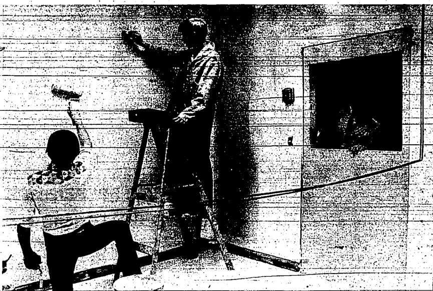
Working on a remodeling project at Stuart Junior High School are Ken Tuma, Thomas Riley and Benny Wright, from left.
