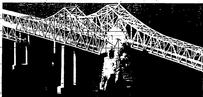
Demolition experts drop a dangerous overhanging fragment of the Sunshine Bridge.
