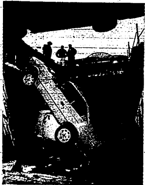
Several cars were damaged when the roof of a parking garage in Seattle collapsed Friday.
