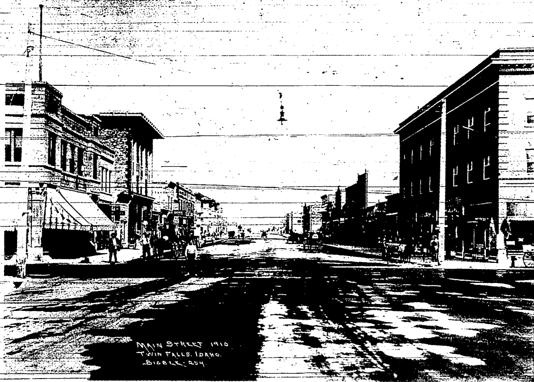
The Idaho Department Store, left, is still in the same location on Twin Falls' Main Street, but transportation was quite different in 1910 when C.E. Bisbee took this photograph. Dime sign at left is for a dime theatre. The Perrine Hotel, long a Twin Falls landmark, can be seen at corner of Main and Shoshone at left rear.
