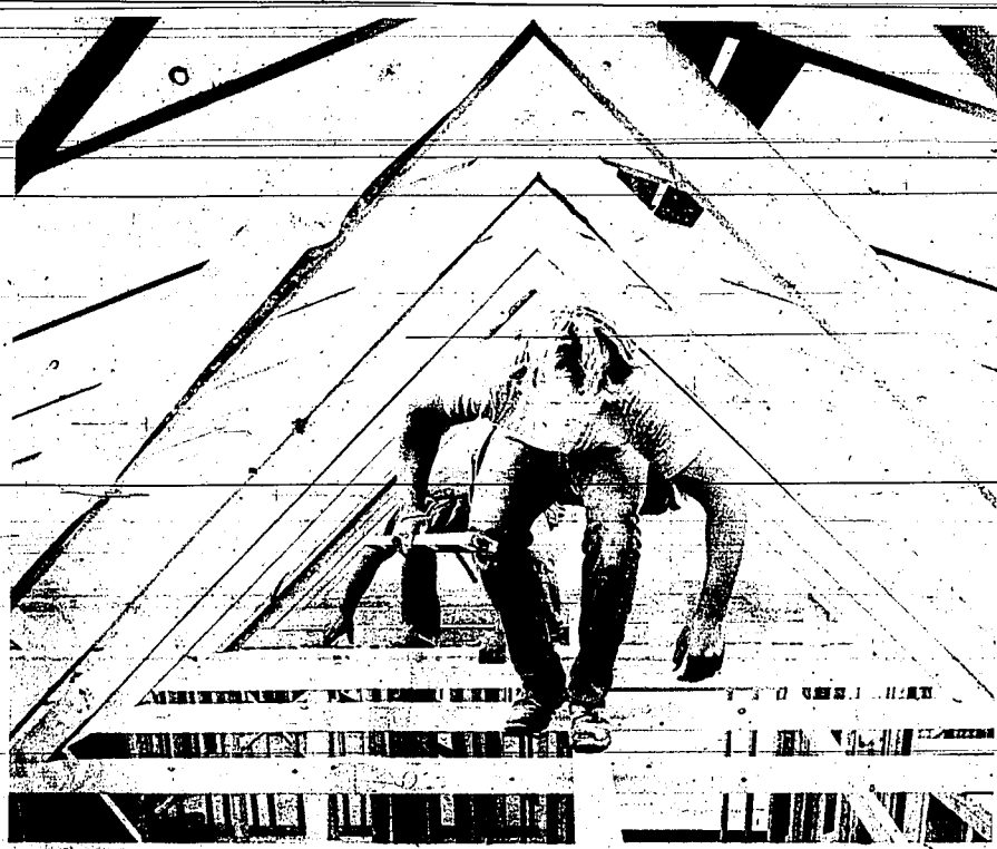
Rain, rain, go away . . . A jigsaw puzzle of roof supports were quickly put in place Monday as carpenter Todd Whitman raced to beat the rain. Work on a duplex at South Park in Twin Falls. Twenty-four buildings, some with two, three and four bedrooms, are 50 percent completed for the Idaho Migrant Council Farm-Labor-Housing Development.
