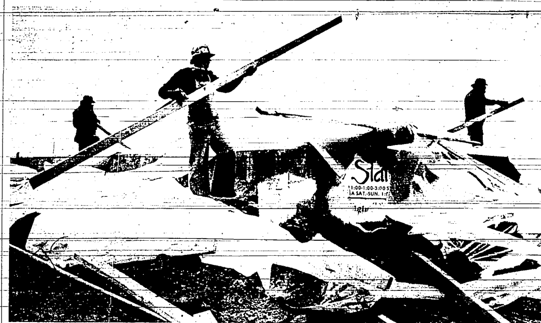
Workmen of the Mid-State Construction Company of Twin Falls played pick-up after 50 mph winds scattered work materials for the new KLIX Building
