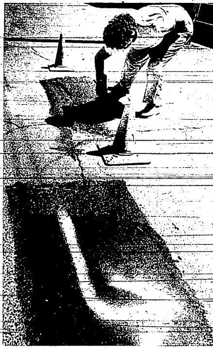
Robbi Dunlap of Twin Falls applies a test asphalt mixture
