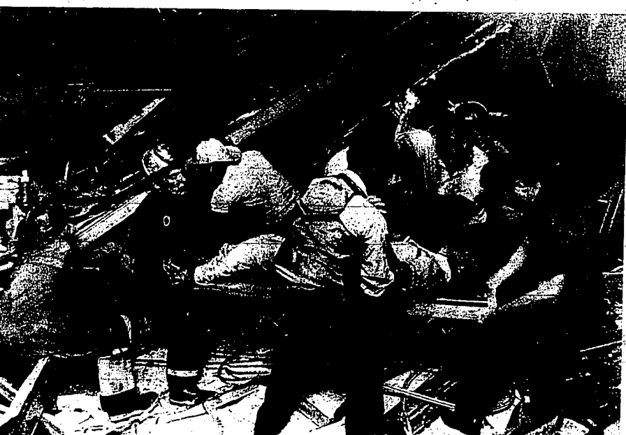
Kansas City rescue crews remove an injured man from under a collapsed walkway in the lobby of the Hyatt Regency Hotel
