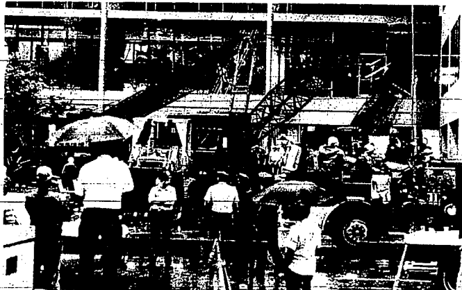
Workers use cranes Saturday to remove the rubble after a walkway collapsed.
