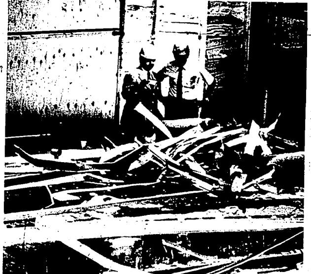
Investigators inspect the crumpled skywalks on the Hyatt Regency Hotel lobby
