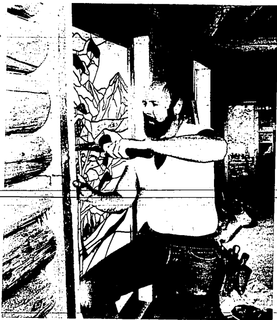
Home builder Stan Stanley installs leaded windows depicting nearby peaks
