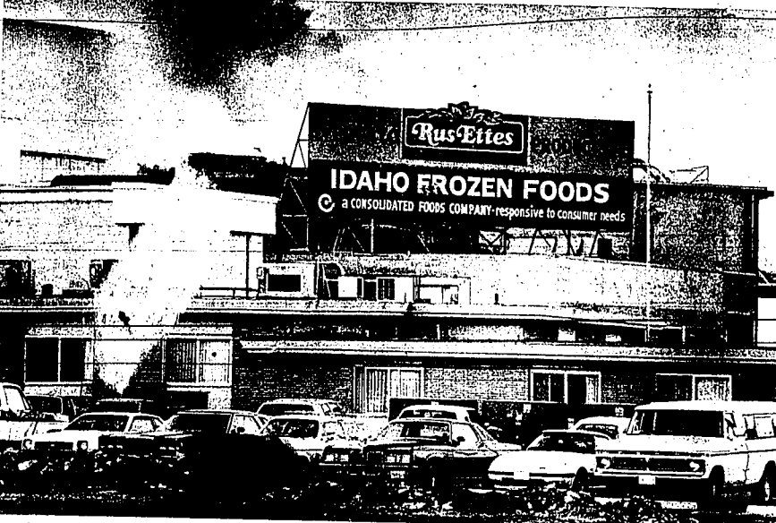
Idaho Frozen Foods awaits authorization for its own sewage treatment plant and will withdraw from the Twin Falls system
