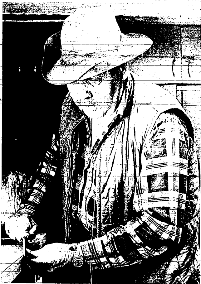
Tom Frith works to smooth a counter top in Dr. Paul Youcum's new office
