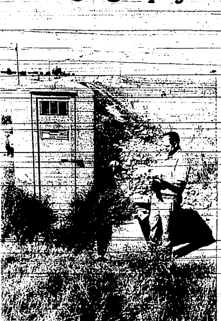
This gravity-fed aquifer recharge system uses river flows
