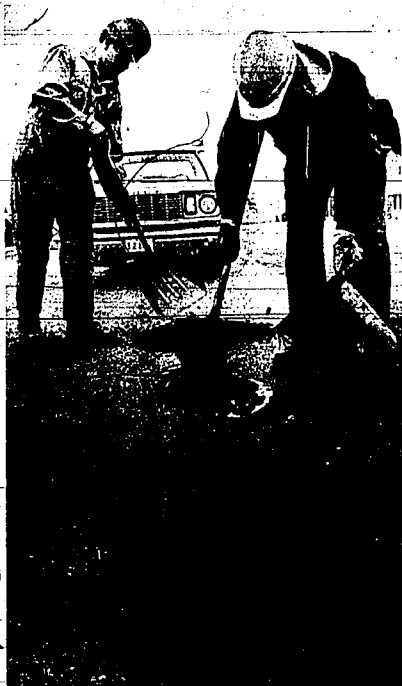
Oil, gravel make temporary pothole patches
