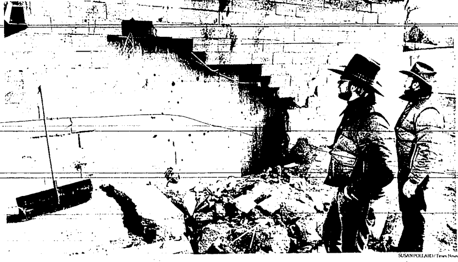
Manager Tom Tarter, left, and president Jim Tarter inspect the damage at their OK Tire store after Wednesday night's explosion
