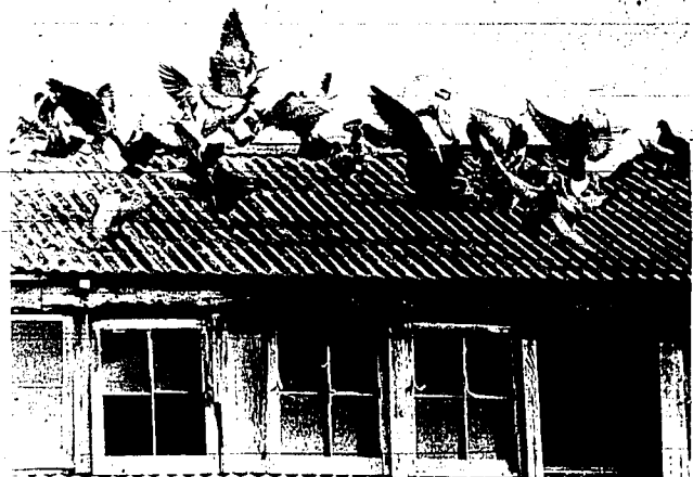
An abandoned warehouse with broken windows provides easy access to a pigeon nesting spot
