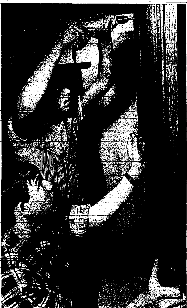
Seniors Mike Etcheverry, back, and Robert Reed add the finishing touches to building
