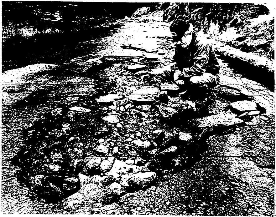
Floyd Dayley of the Twin Falls Highway District evaluates the damage on Shoshone Falls Road on Wednesday.
