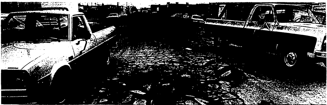
Heavy semi-trailer traffic on Third Avenue West first rippled, then crumbled the winter-softened pavement. Drivers traveling along Third found progress slow.
