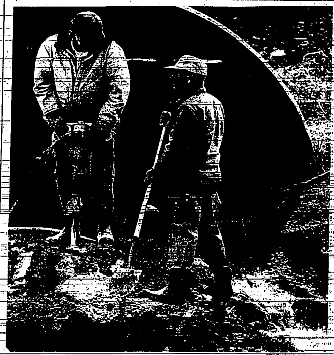
Chipping away Floyd Swan, left, and Ed Newman of the Twin Falls Water Department chip away a slab of concrete below the Eighth Avenue lateral. The men were clearing the concrete to allow the water to flow better when the city's canals are opened, possibly later this month.
