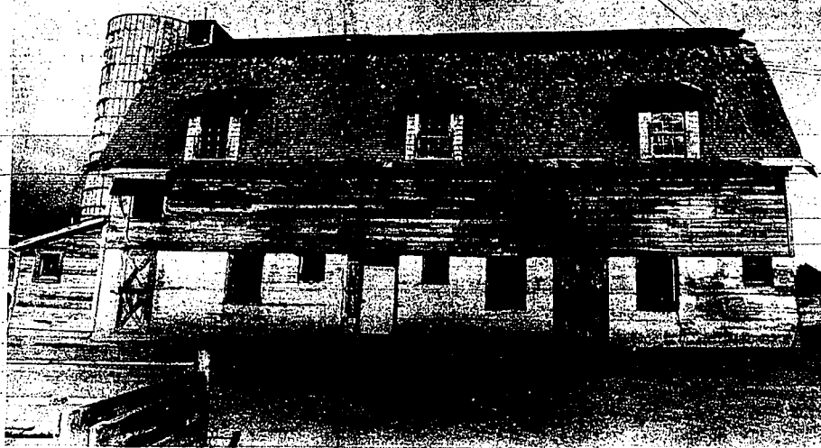
Built for Art Maxwell in about 1908, this barn off state Highway 30 contained a cloak room for use during barn dances
