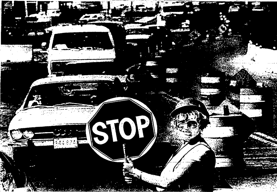
Cindy Charlton directs traffic as construction crews continue work on Blue Lakes Boulevard
