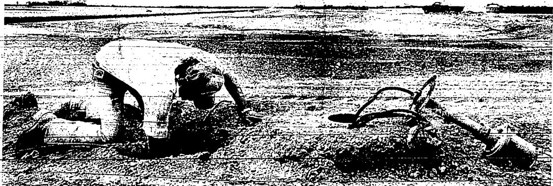
Fred Brower from Bengal Electric in Pocatello rewires airport lights at the end of the 7,150-foot runway which is being extended to 8,700 feet
