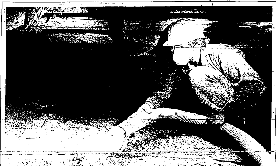
Insulation consisting of fire retardant ground-up newspapers and cardboard is sprayed into an attic by Ruben Salazar.
