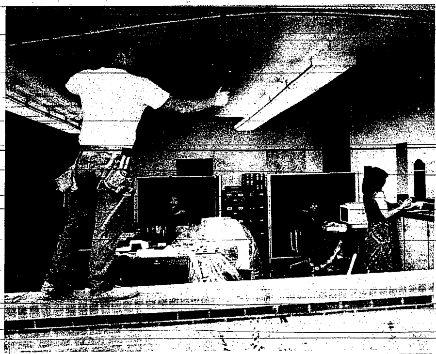
Office workers at Twin Falls City Hall had unusual "air conditioning" Thursday, as Malcolm Emery installed a new window.
