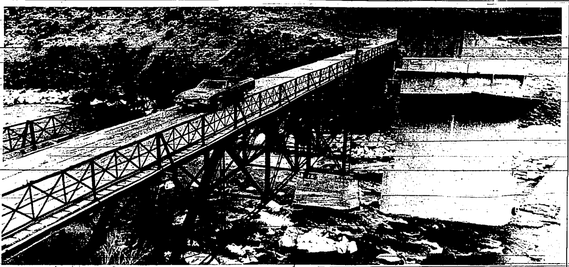
A car snakes its way over the old bridge near Murtaugh, past the concrete abutments which will support the new bridge when it finally is completed.
