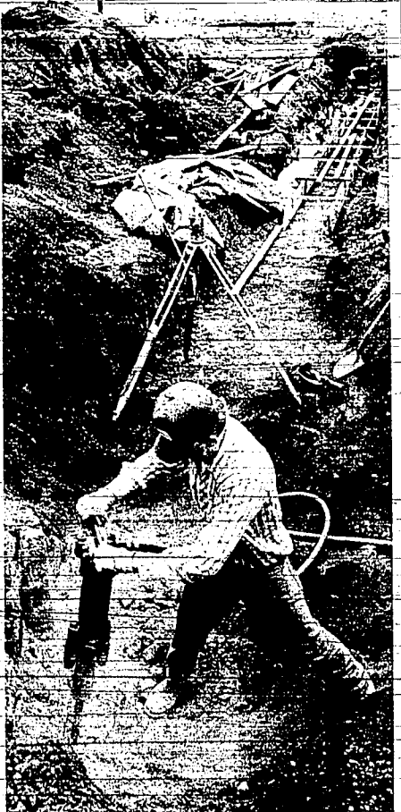
Highway crews work on approaches to bridges
