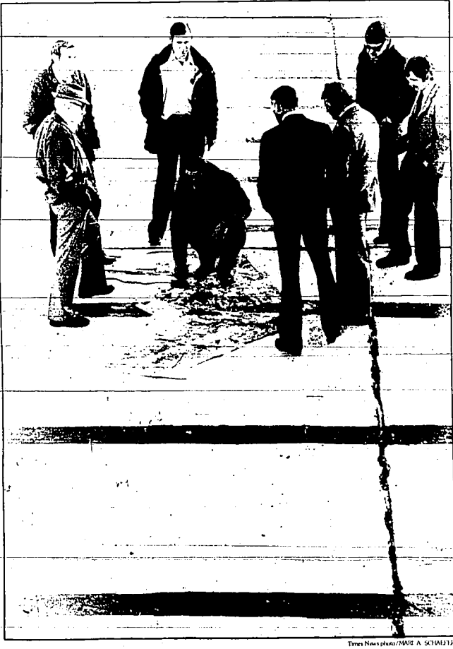
Twin Falls City Council toured Harmon Park Pool to inspect damage and decide its future
