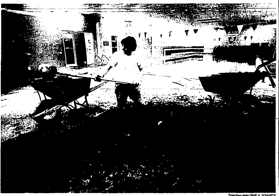
Alton Henry of Wendell was one of the workers digging out a hole for the Y's new hot tub Thursday
