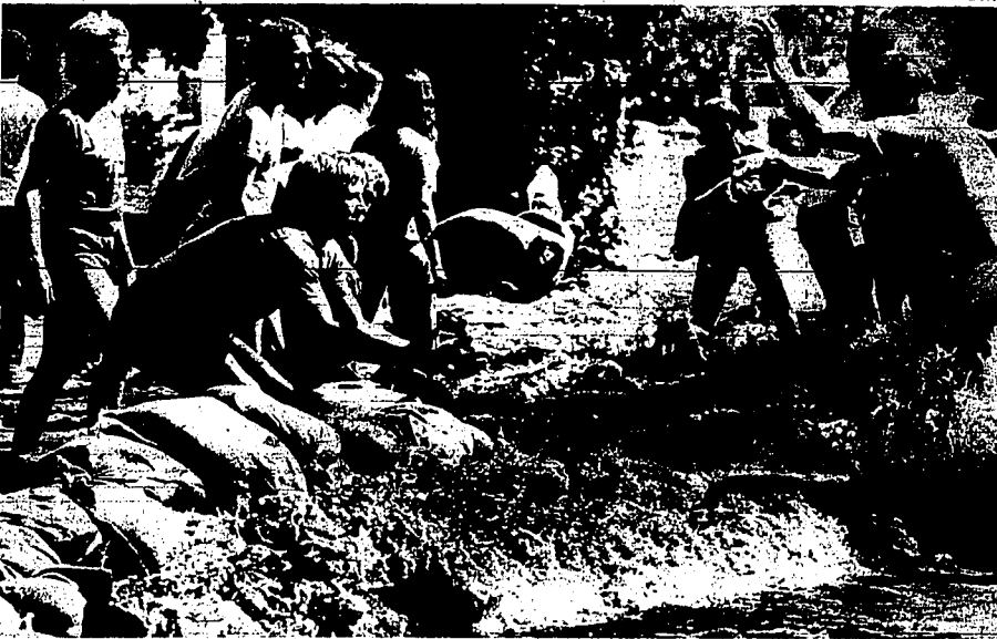
Volunteers battle to build sandbag dike Sunday in Salt Lake City's Memory Grove, menaced by overflowing City Creek
