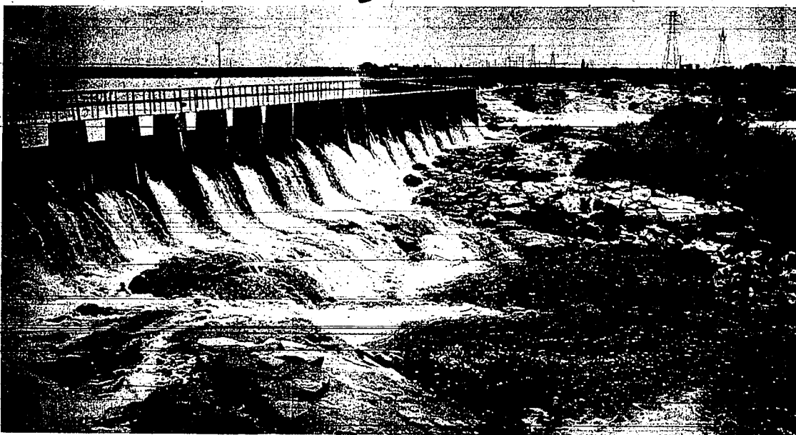
The Minidoka Dam power plant, with five turbines, was built in 1908 and is the oldest public hydroelectric project in the Pacific Northwest.
