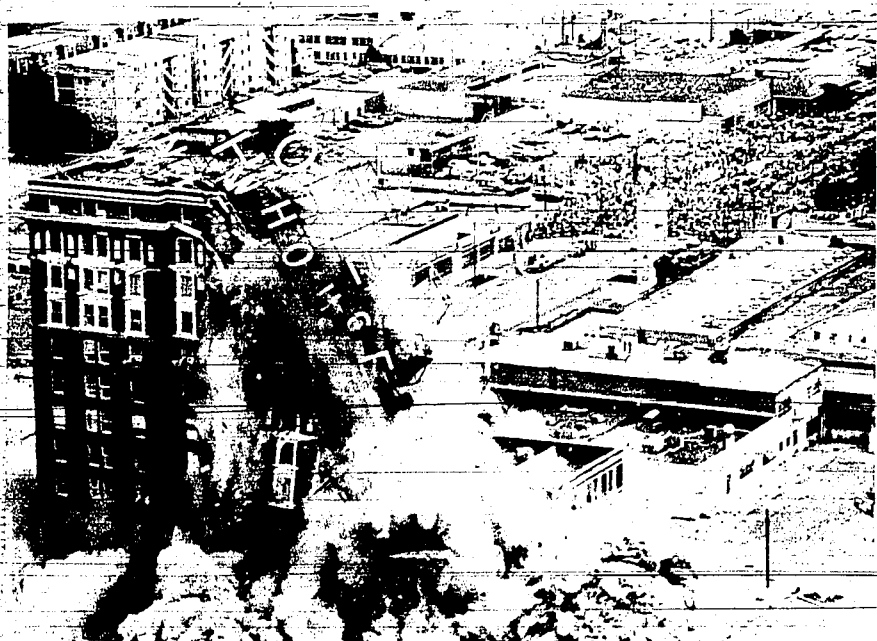
Newhouse Hotel in downtown Salt Lake City begins to crumble as large crowd watches explosives sever its steel frame
