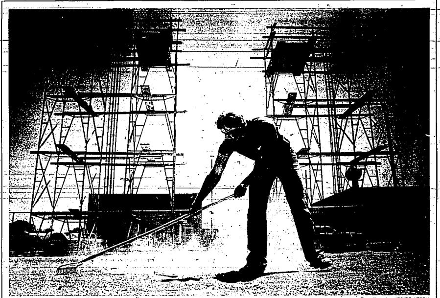
Raking money Bret Judy, of the Judy Co. of Boise smoothed gravel over a vapor barrier of Folse in preparation for laying the foundation for the new Idaho First National Bank building in downtown Twin Falls. The building, at Shoshone Street and Third Avenue North, will replace the present offices at 103 Main Ave. E. It is expected to be completed by early 1984. The CM Co. of Boise is the general contractor.
