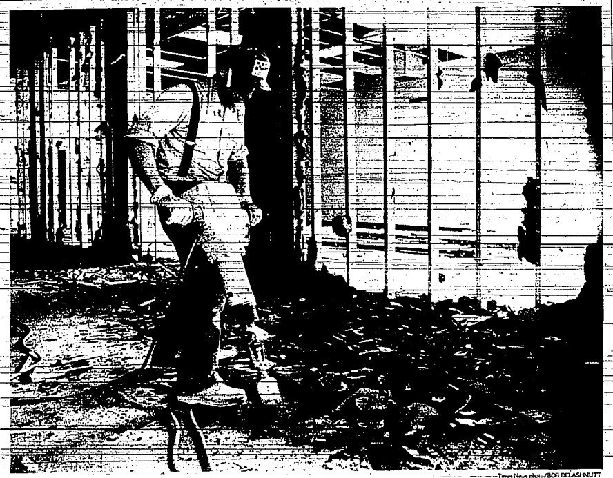
Stubborn floor John Hall of Armstrong and Co. blasted away Monday at the stubborn asphalt on the floor of the Old Times-News building. The structure is undergoing remodeling and will provide new office space for the downtown area. The project will be completed in early 1984.
