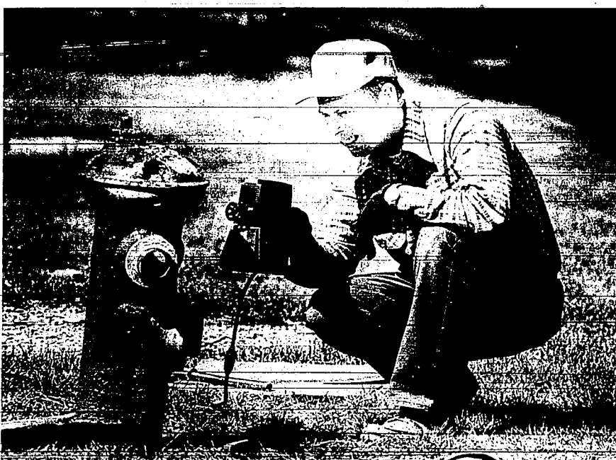
Water department worker Richard Jones sprays a coat of red paint onto a hydrant at Seventh Avenue and Fourth Street
