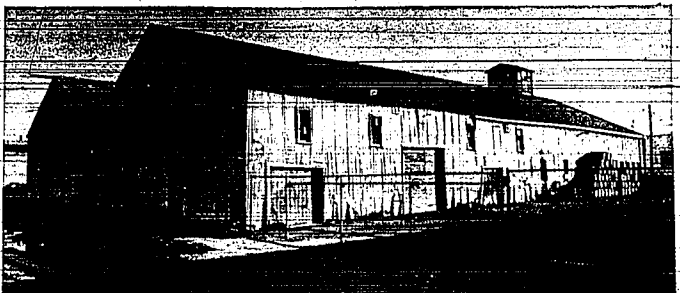
Two Jerome farmers say they can't get $5,000 worth of their beans out of this warehouse
