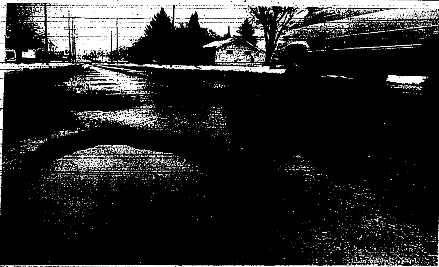
It's a pothole season again: Workers will patch monsters like this one on Filer Avenue West in Twin Falls as soon as possible.
