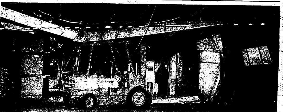
A workman peers into the collapsed structure at Conida. Much of the roof was prevented from falling further when it hit a parked forklift
