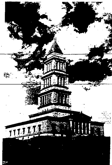
George Washington Masonic National Memorial Building
