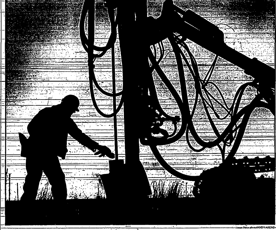
Getting ready to drill Ed Crumrine, of Western Construction, tends to his air-track drill while making holes for blasting charges in the median along Interstate 84 near Jerome. Crumrine is part of a crew busy leveling outcrops of rock in the median. The project is aimed to enhance safety along the Interstate.
