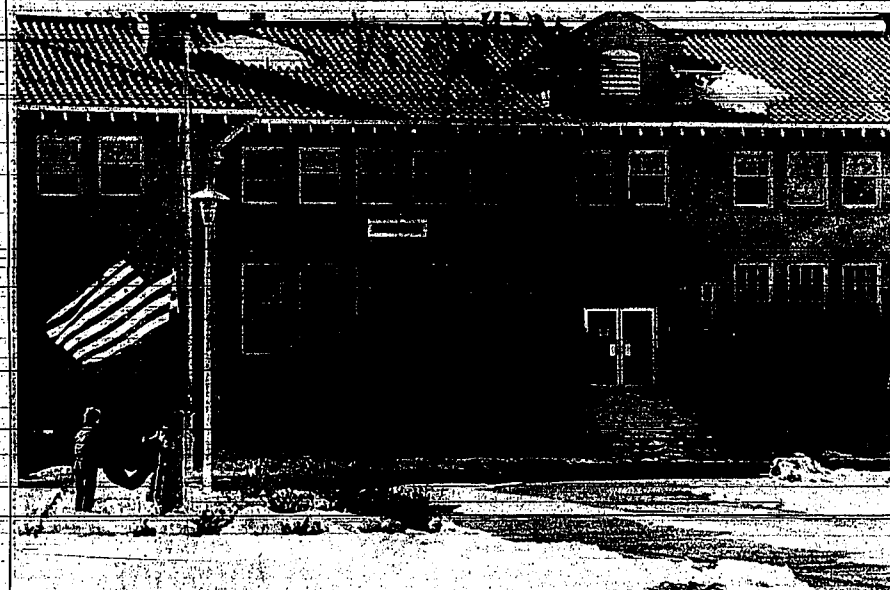
The days of seeing flags folded are limited for a campus building dating back to 1912, as plans are made to level it.
