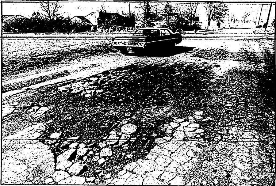
Not only Dodges are dodging potholes on county roads, this Plymouth goes around the broken blacktop of East 3300
