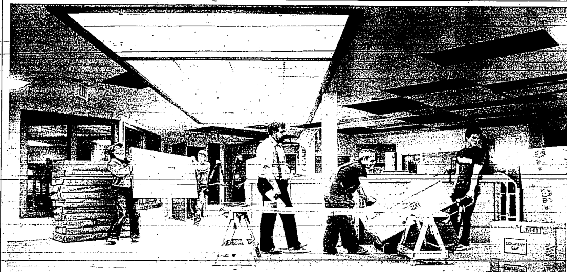
Work is nearly finished on Canyon View Hospital, the new Heritage Health Care Corp. hospital being built on Shoup Avenue West in Twin Falls
