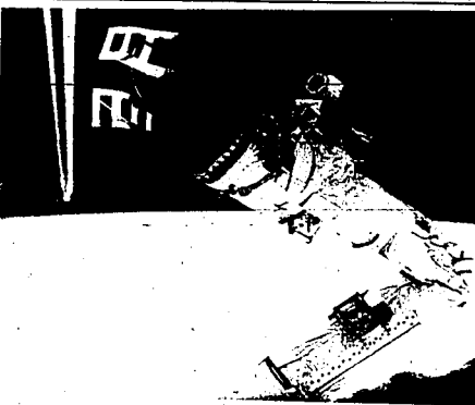
Broken swatters at end of effector device was one problem
