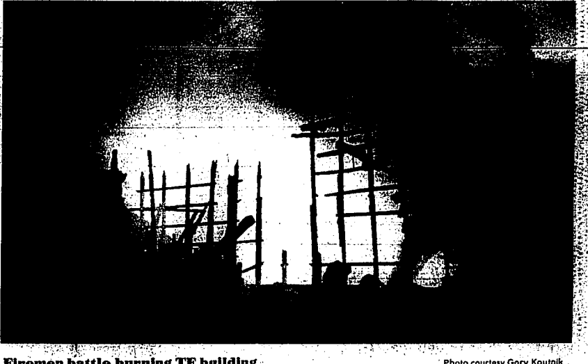
Firemen battle burning TF building
